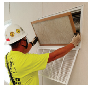
Figure 6 Remove old filter
