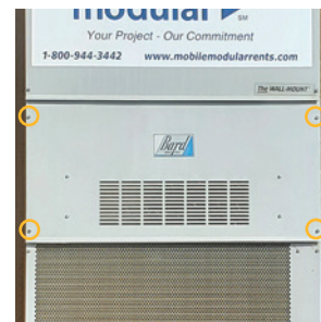
Figure 3 Outer screws location
