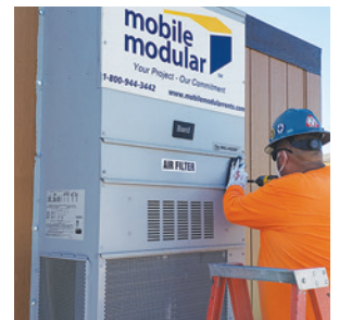
Figure 4 Remove old filter
