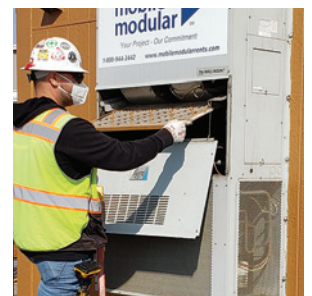
Figure 4 Remove old filter
